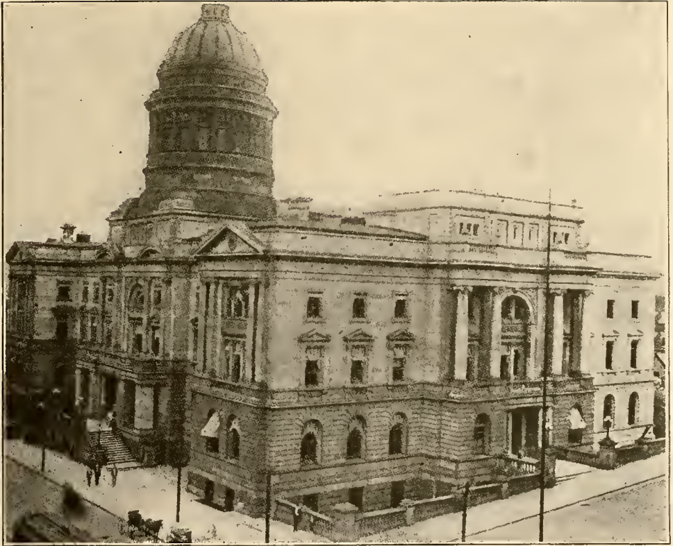
NEW FEDERAL BUILDING.
